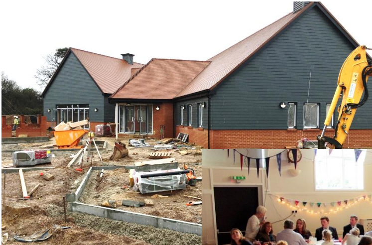
Abbotswood Community Centre, fitting out a new build
