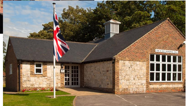
Southwick and Widley D-Day Memorial Hall, new doors and windows
